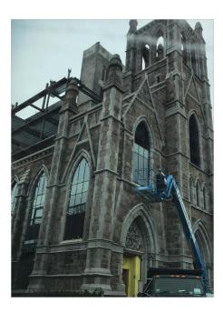
Several years ago, Lawton Welding, a miscellaneous metals and small structural steel company based in Topsfield, Massachusetts, took on a project detailing and fabricating the steelwork for an old stone church that was being renovated and repurposed. The project was fraught with rework orders – largely due to the irregularities of the stone structure – and took nearly three months to complete.
